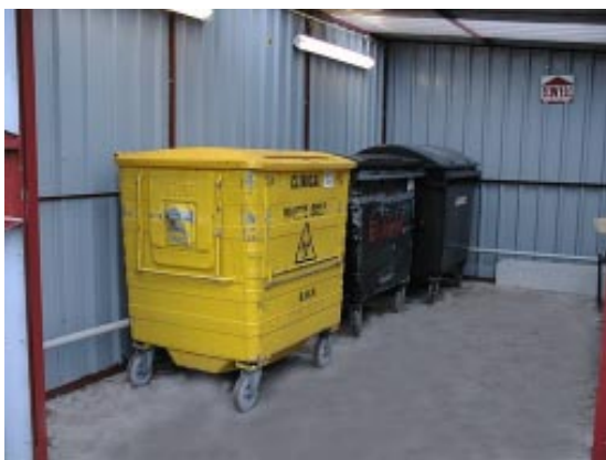
Building detailed 3.66m width x 5.59m length x 2.2m to 2.59m height, single 1.50m door. Terracotta plastisol cladding. Rain water goods & roof light panels
